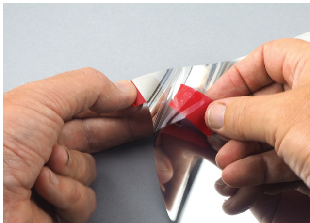
Figure 3-14: Removing the plastic backing from the reflective window film
