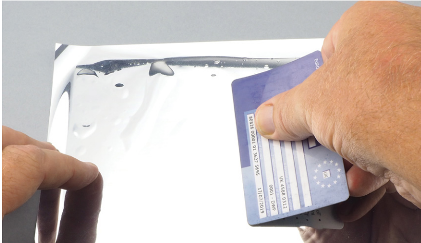
Figure 3-15: Removing bubbles from the reflective window film
