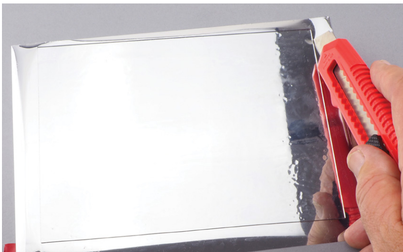
Figure 3-16: Trimming the reflective window film
